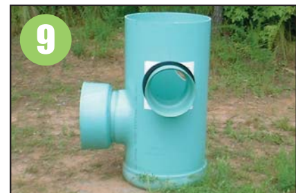
9 Add-a-Branch installation is complete and ready for pipe to be inserted.
