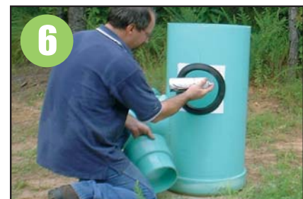
6 Once the Add-a-Branch gasket is installed, lubricate inner surface with standard pipe lubricant.
