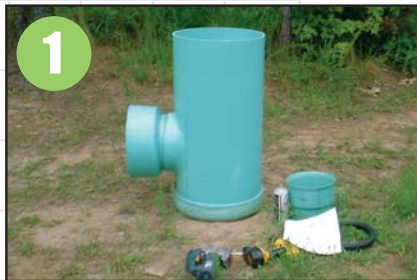
1 Nyloplast Drain Basin ready for Add-a-Branch Installation.
