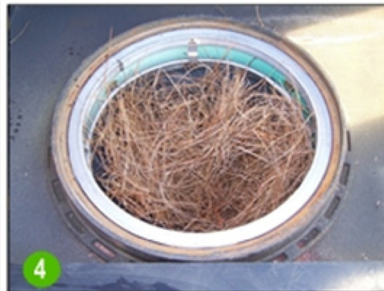
4 To clean the Catch-It™ remove the grate
