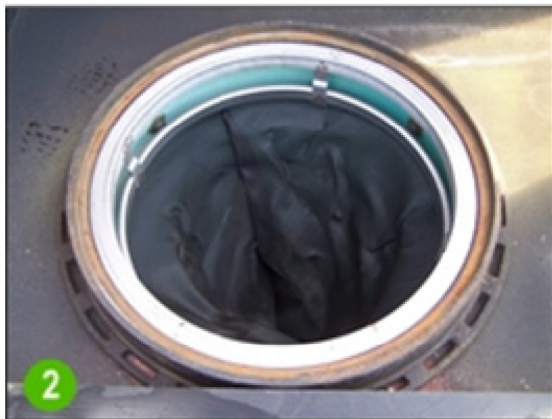
2 Clean debris from frame and install Catch-It™. Check for proper fit
