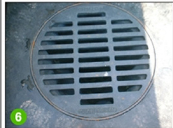
6 Reinstall the grate for safety while emptying the Catch-It™ then repeat the installation
