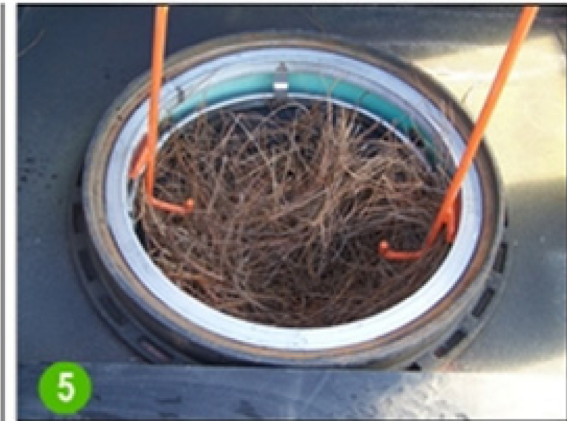
5 Using the FLEXSTORM Universal Removal Tool or other lifting device lift the Catch-It™ straight up
