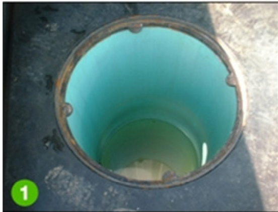
1 Nyloplast drainage structure & frame (24" shown) ready for FLEXSTORM Catch-It™ install
